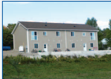
The new St. Peter and St. Paul double residence, completed this summer.
